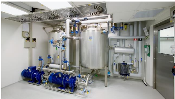
Figure 1. Clean in Place System [1]
